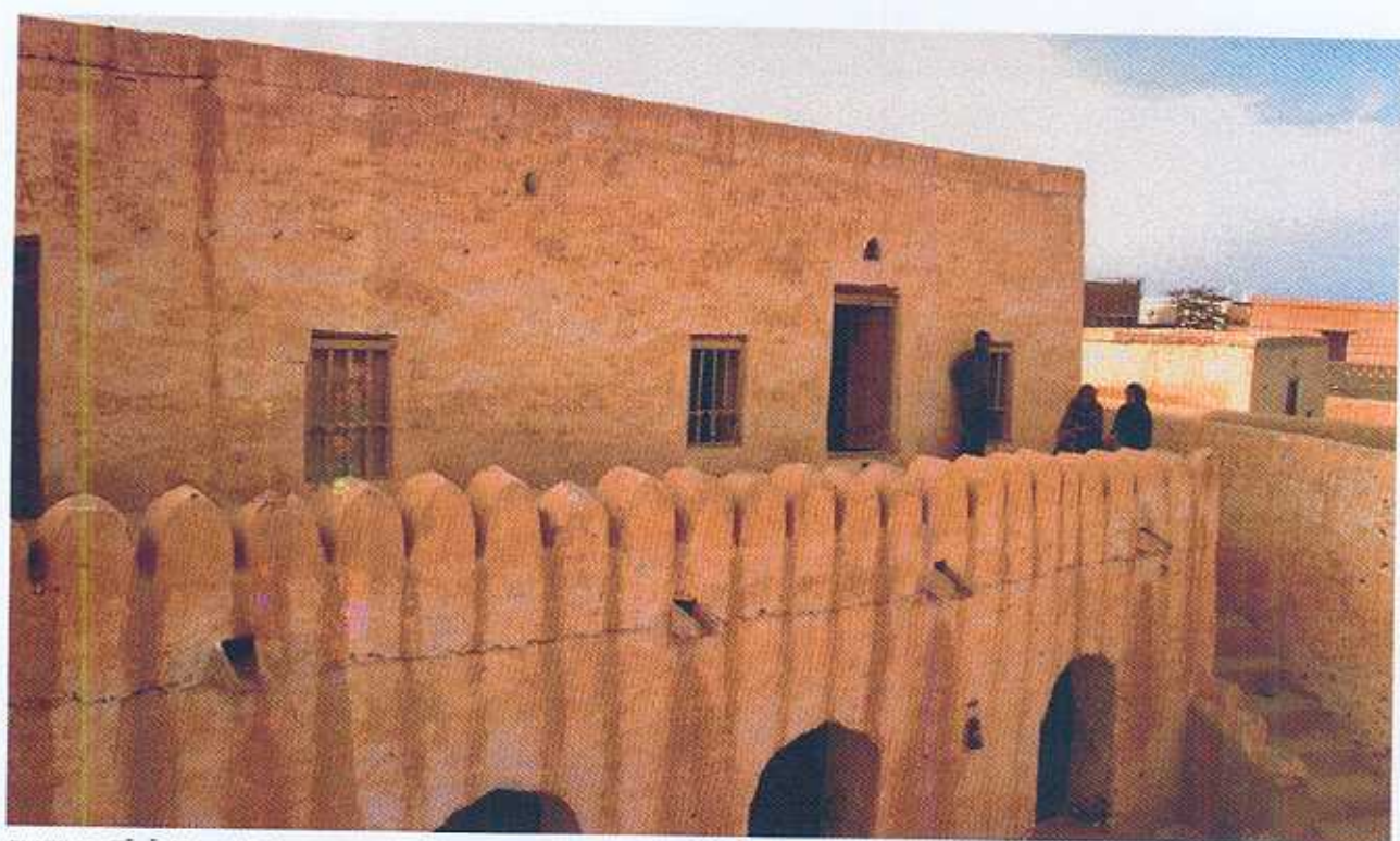
PLATE 17. Īwī, House VI. Courtyard view from S.
