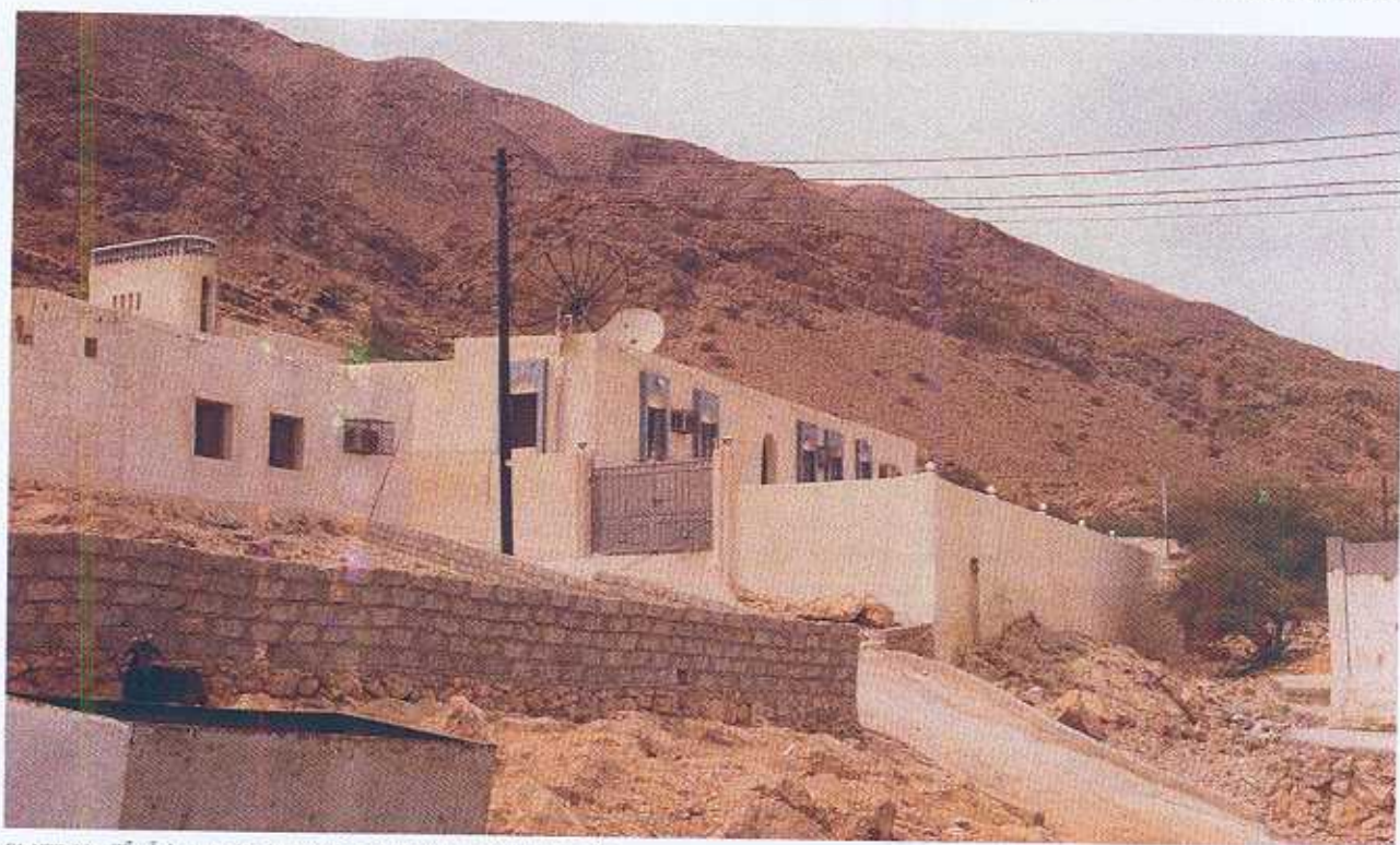
PLATE 22. Ṭīwī, houses in the new residential area. View from SE.
